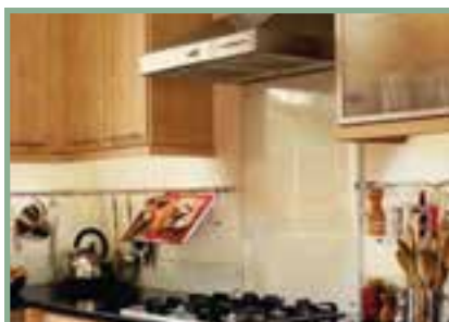
Installation photo employs TaskWork 120V Modular under each cabinet section.
