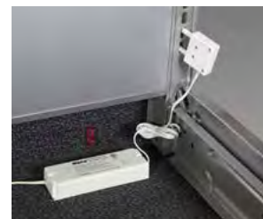
Step Four: Plug Power Terminal into gondola and driver into outlet
