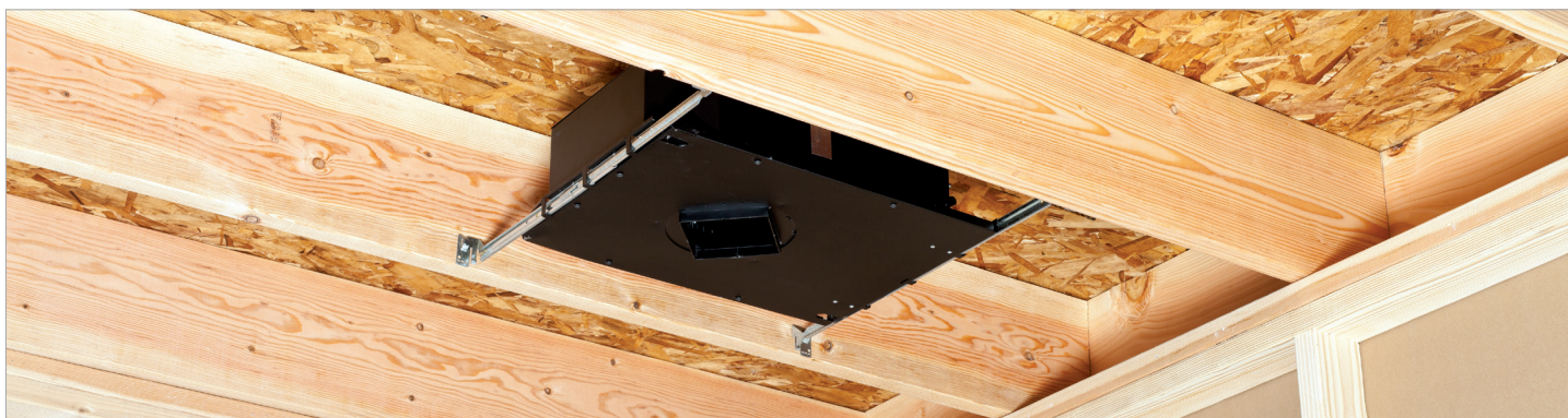
Install housing to the ceiling joists with the adjustable steel hanger bars
