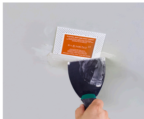
Sheet-metal 3" thin mud plate (optional)
