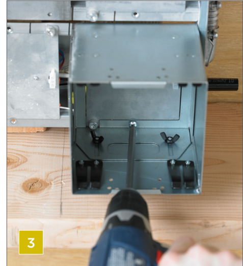
Install housings with screws provided
