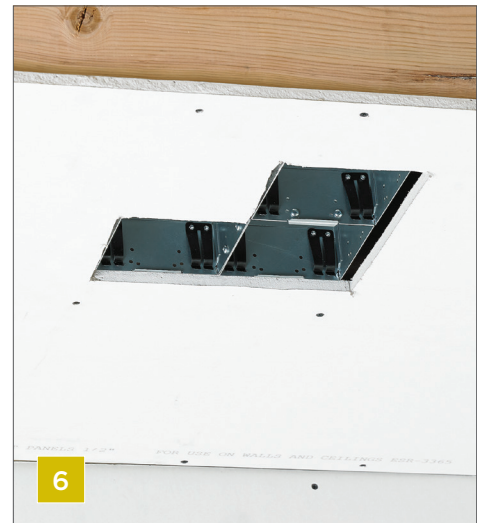
Mount wall board to ceiling outlining the light array design
