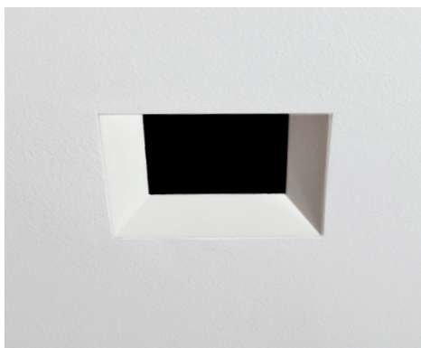
Sand and paint ceiling, then insert flangeless trim
