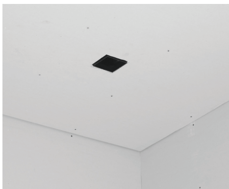
Mount wall board to ceiling and walls
