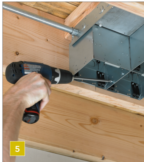
Connect adjacent housings with screws provided
